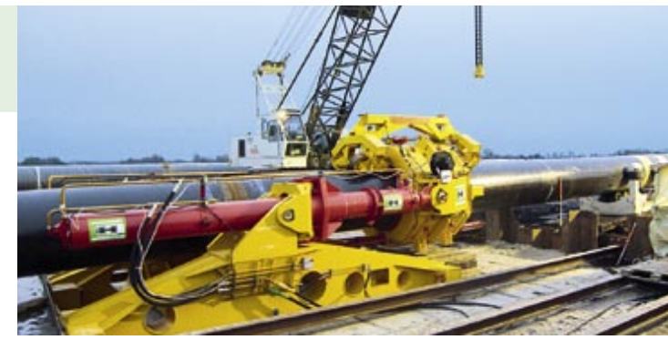
Additional thrust and pulling force for pipe installation with the Pipe Thruster.
